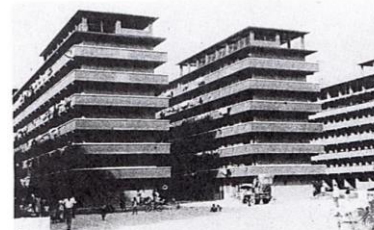
The building upon which the Rooftop project is built. This one building shelters over 3,000 persons. It is one of 22 such buildings in the Wong Tai Sin Resettlement Estate. The penthouse on each end of the building is 70 feet long by 30 feet wide.
